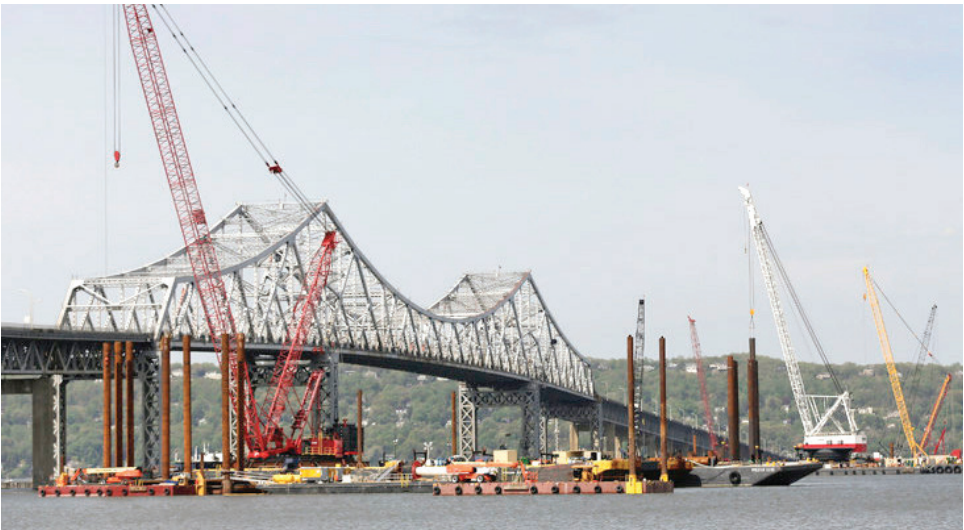
Construction crews use barges and cranes to repair the Tappan Zee Bridge.
